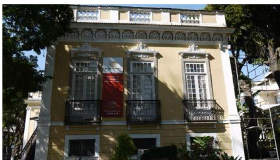
Main exhibition building (currently under refurbishment)
